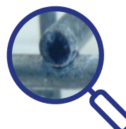
Blackening on the end of the wire
